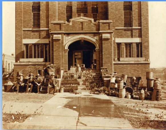
Smith County Jail 110 South Spring Constructed in 1916, in use during the 1930s
