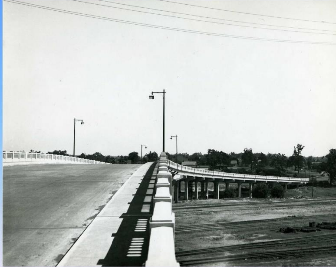
Beckham Street Viaduct 1937
