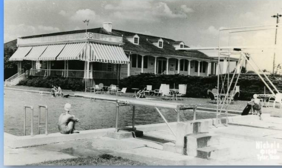
Willow Brook Country Club Swimming Pool constructed 1934
