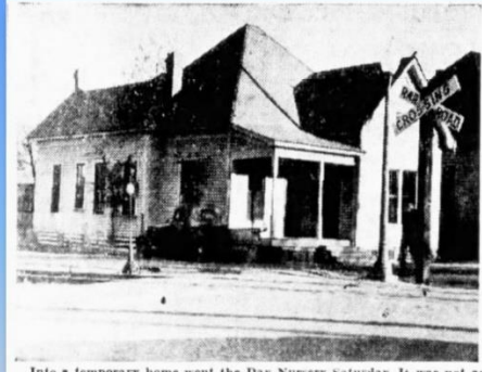
Into a temporary home went the Day Nursery Saturday. It was not as nice as the old, from which the children were forced to move to make way for a new city hall. The house is so close to the railroad tracks at 407 North Bois d'Arc that another assistant is required to watch children at play. The board of directors of the nursery has been given another lot by the city, but as yet there are no funds to build a permanent day home for Tommy and many such like him.—Kenneth Gunn.
