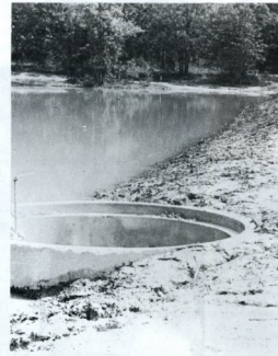
Dangers come in many forms and shapes. One danger at Texas Eastern is a large uncovered pipe with a potential for causing a terrible accident for someone unaware of its existence. This open pipe is located on the west dam of the Texas Eastern lake. Something needs to be done to prevent this possibly dangerous situation from becoming a tragedy. In the darkness this hazard might not be seen by some youngster riding his bicycle along the dam, or by some not very alert student.
