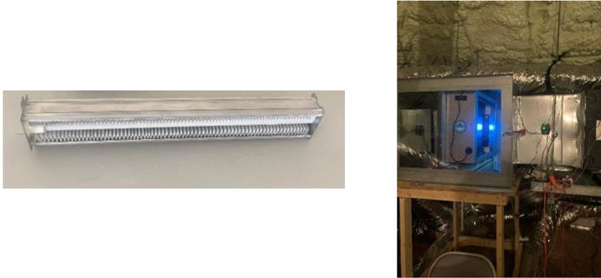
Figure 32. PCO B core (left) and in plenum (right)
