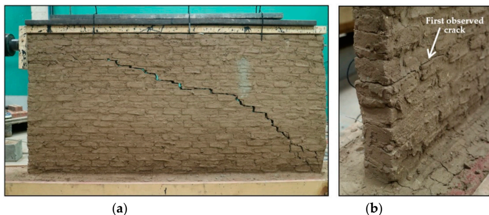
Figure 9. Wall 2: (a) near failure; (b) first crack at the transition between wet and dry regions.
