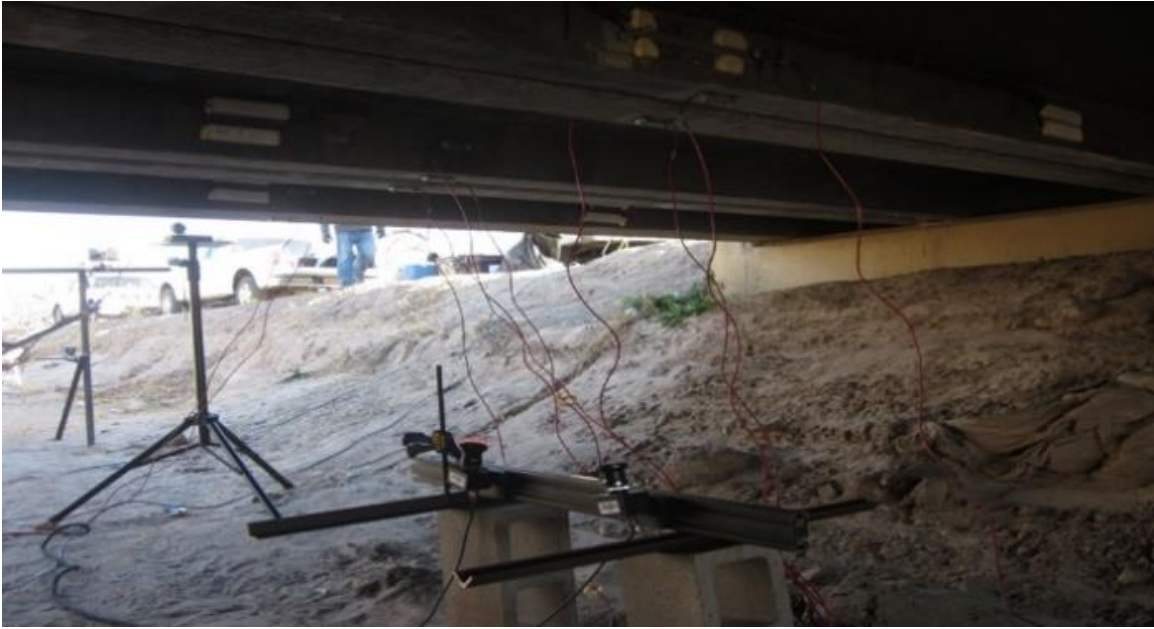
Figure 10. 2M System for monitoring an interior girder of UHPC span
