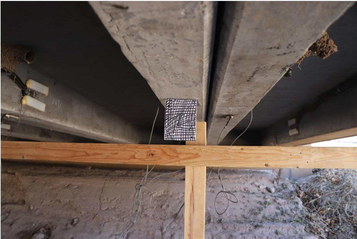
Figure 17. Internal girders with attached targets for displacement measurement
