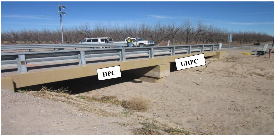
Figure 1. Bridge test structure
