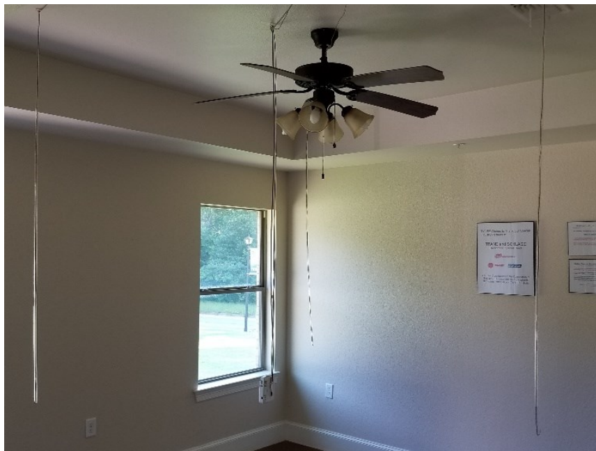
Figure B4. Master bedroom
