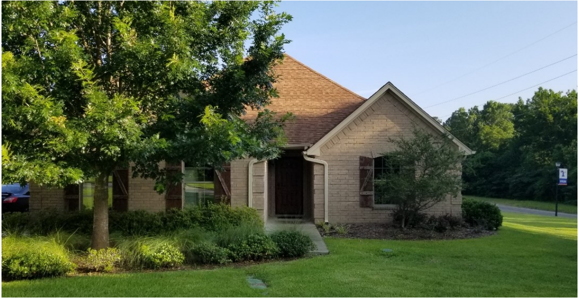
Figure A3. Front of VRF ducted-ductless HVAC system house
