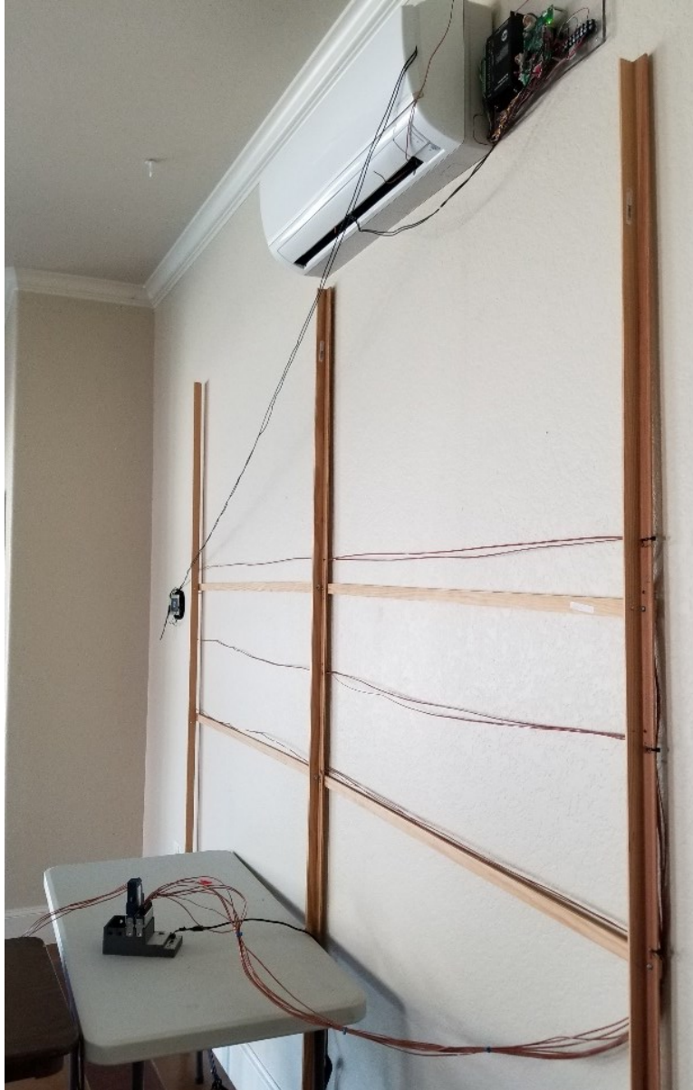
Figure B8. HW3 in living room with temperature grid on wall
