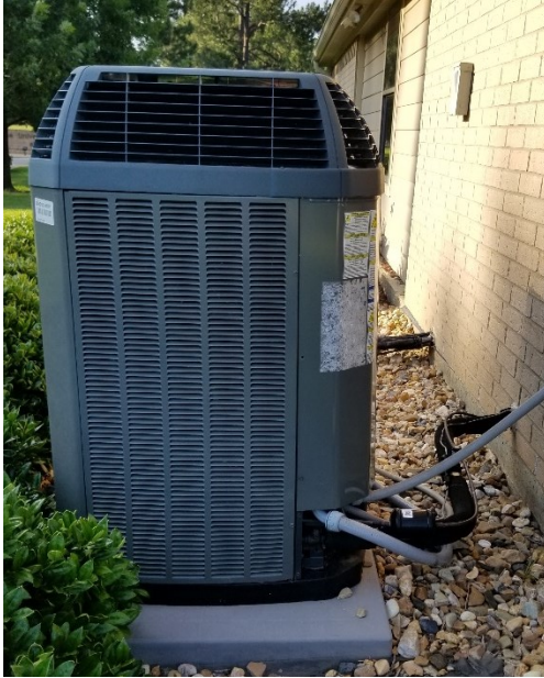
Figure 6. 3-ton outdoor unit
